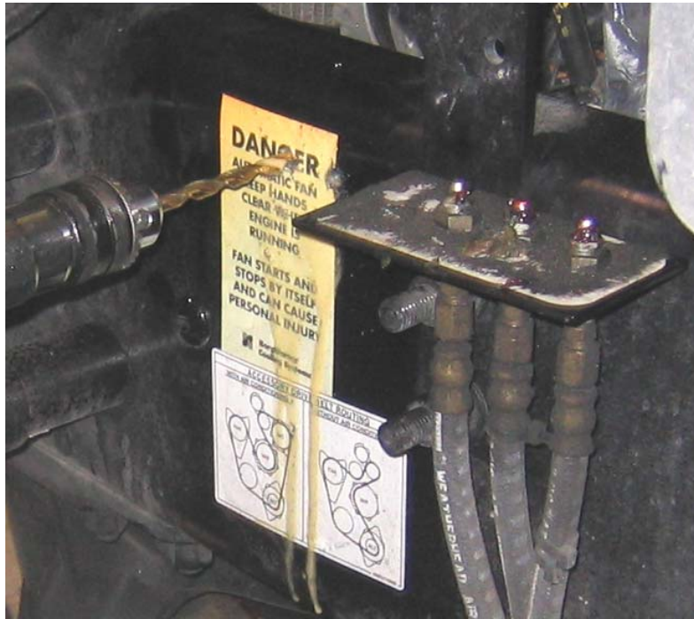
Figure 4 – Drilling the Mounting Holes for the Filter
